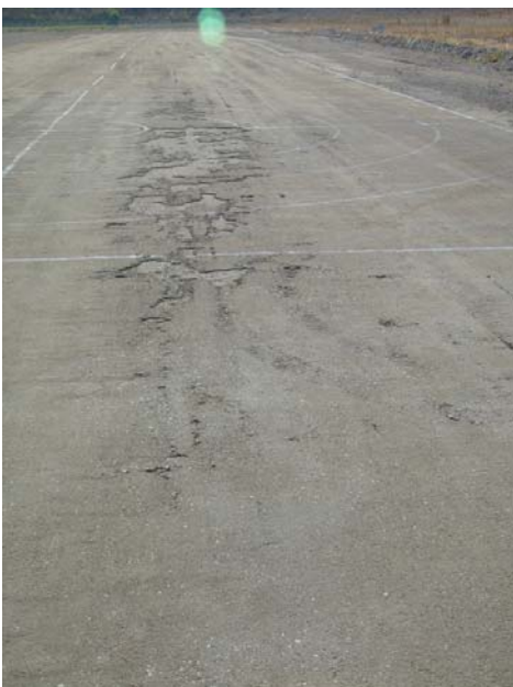
Runway center section looking from East to West—After removing all debris
